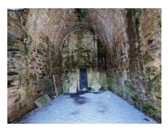
The sandstone that was primarily used for the construction of the chapel has been significantly damaged by moisture. To save its frescoes, extensive restoration and preservation work is being done and dehumidifiers are installed to dry out the stone. The chapel is only open for limited guided tours and you should call ahead to understand when those tours are.
